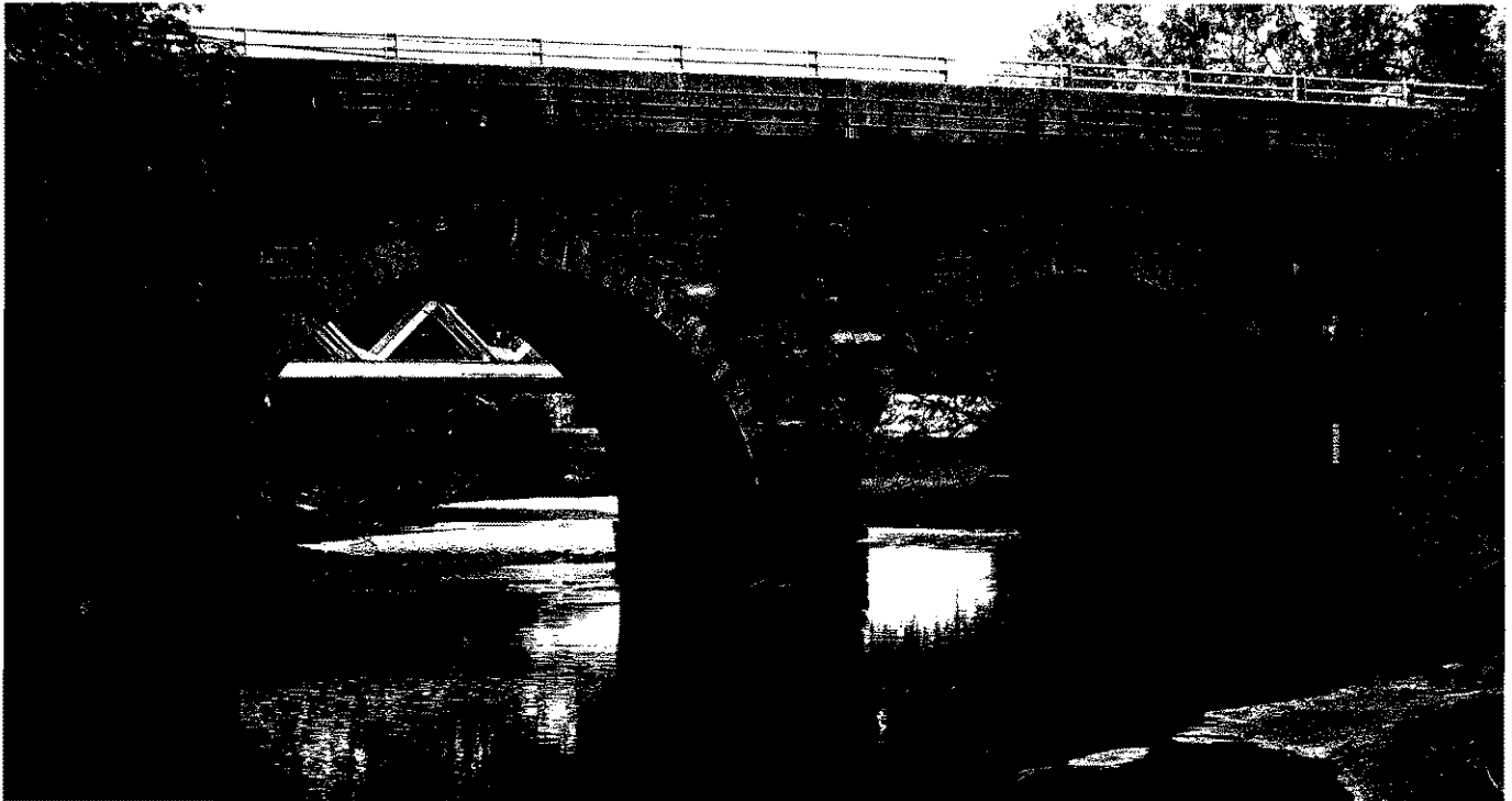
The historic State Street Bridge (c. 1848) erected over the Rippowam (aka Mill) River to carry the newly-constructed railroad from New York City has untapped potential to create the kind of vibrant urban experiences millennials and boomers look for in downtowns.
