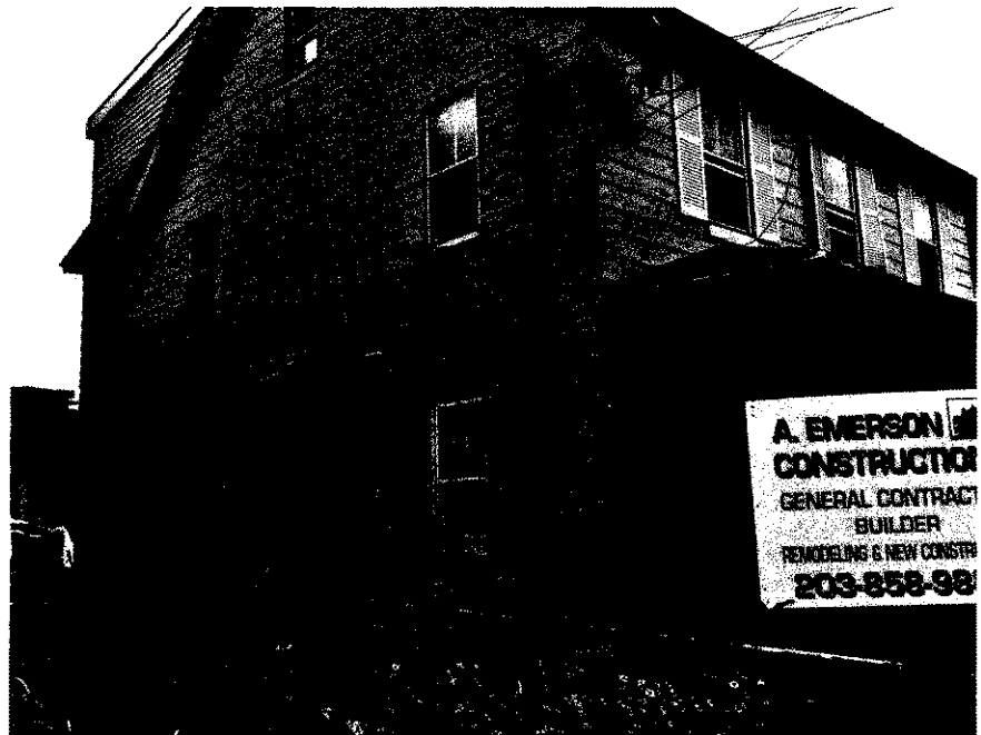
38 Ann Street prior to rehabilitation
