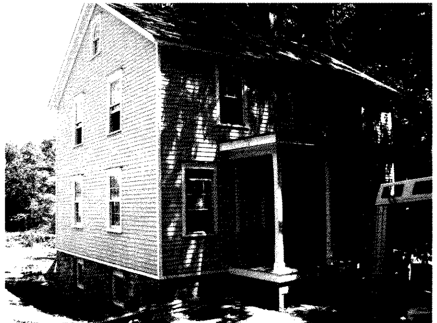
Rebuilt parsonage nears completion
